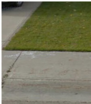
This would pass inspection
