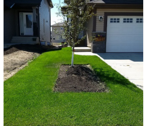
Area around tree is unfinished
